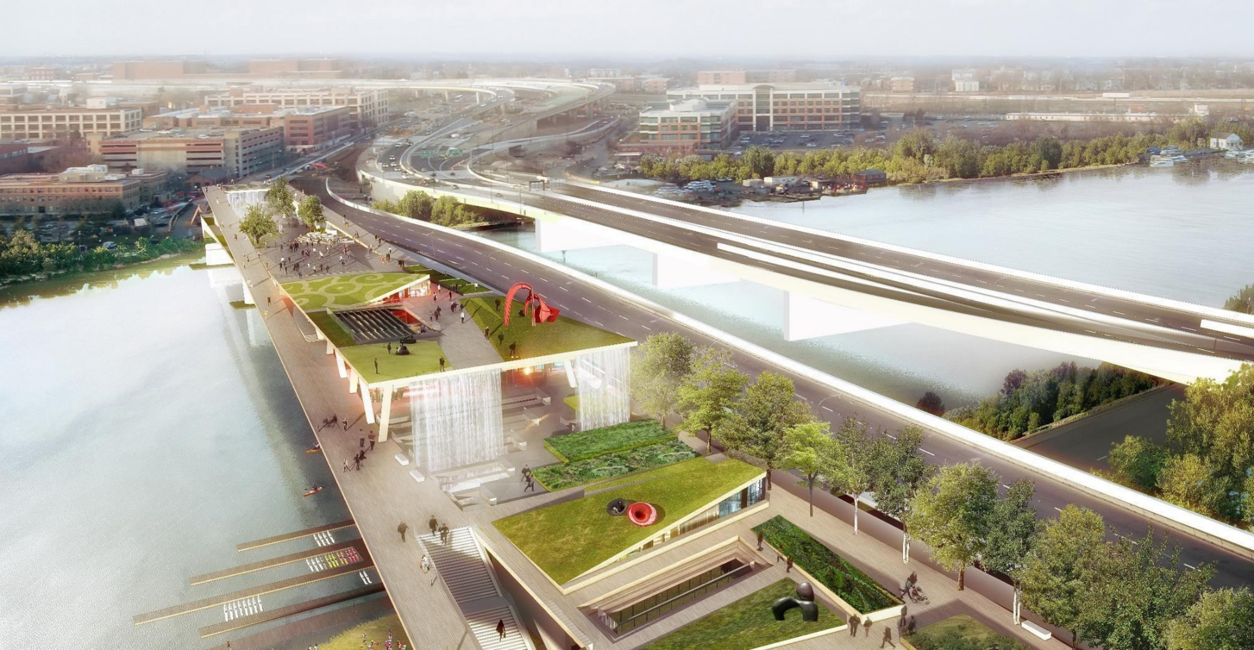
11 th Street Bridge Park, Washington, DC
