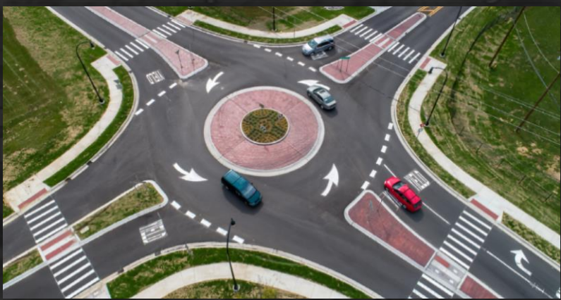
New Roundabout at 6 th Ave w/ adjacent shared use path to accommodate cyclists
