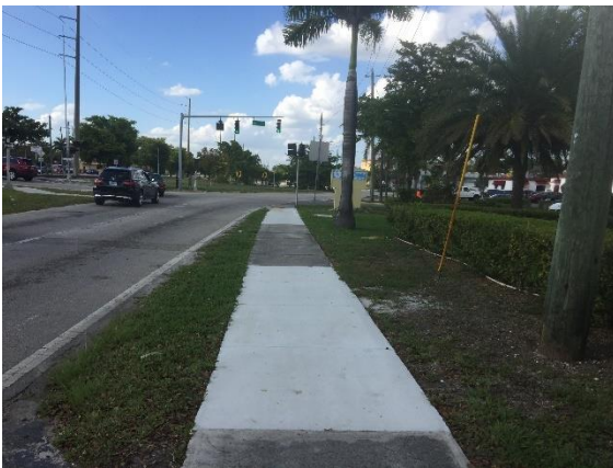
Sidewalk on the east side of SE 1 st Avenue with a buffer between the sidewalk and curb, also known as a furnishing zone.
