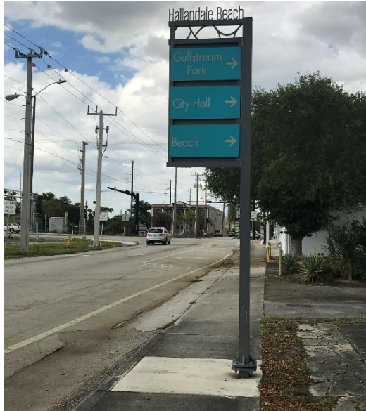
The wayfinding signage is being held with a breakaway base support. Breakaway base support can reduce damage to cars and occupants.
