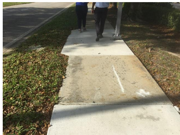
The wayfinding signage is properly installed to provide an unobstructed pedestrian zone.
