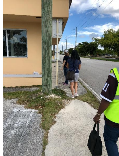
Unmaintained landscape encroaches the sidewalk facilities.
