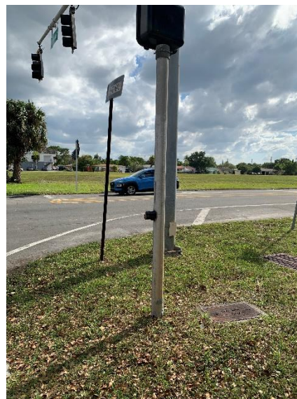
The pedestrian signal and pedestrian pushbutton is located in the northwest corner of Dixie Highway and SE 3 rd Street without providing a clear and accessible path for non-motorized users.
