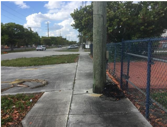
Street fixtures are within the sidewalk, which prevents a clear pedestrian zone and utility cords have not been properly placed.
