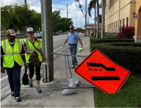
Construction signage knocked down in front of 134 S Dixie Highway.
