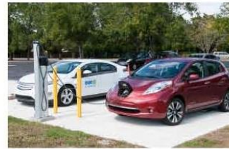
Electric Vehicle Parking & Charge Stations
