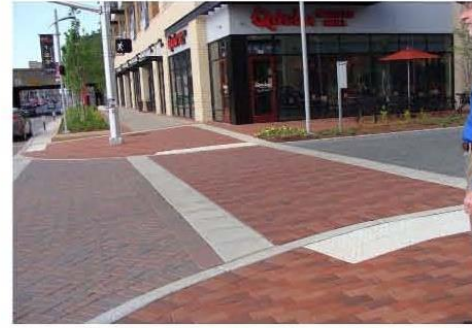
Raised Pedestrian Crosswalk
