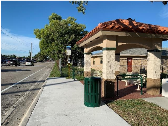
Route 31 – Stop ID# 2646 at the northeast corner of NW 31 st Avenue and NW 39 th Street includes amenities that should be emulated along the corridor such as benches, trash receptacle, bike racks, and a handrail.
