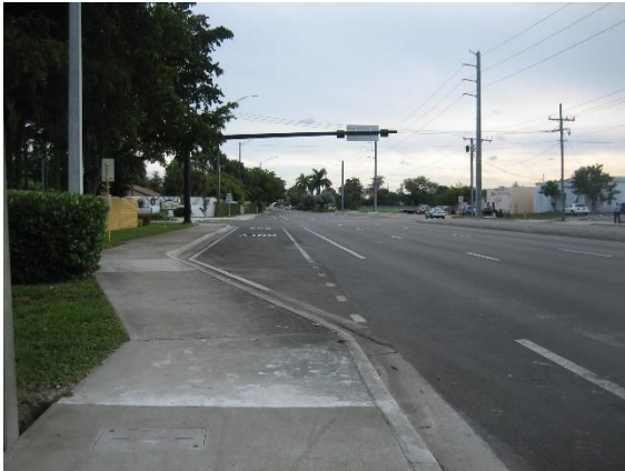
Dedicated bus bay Route 31 – Stop ID# 2644.
