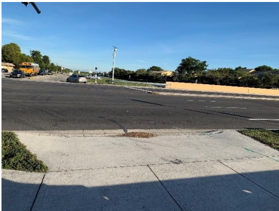
Provide a marked crosswalk with detectable warnings on curb ramps at NW 31 st Avenue and NW 39 th Street for the southern leg.
