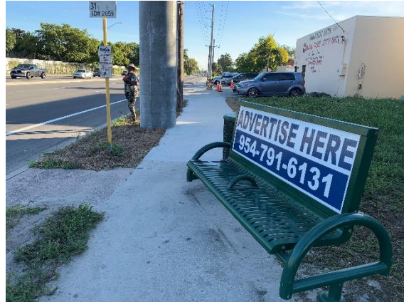
Route 31 – Stop ID# 2659 does not have proper ADA landing pad/passenger waiting area or pedestrian lighting.
