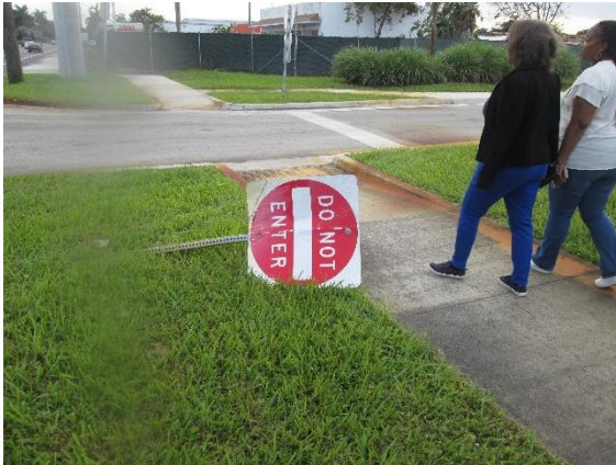
The MUTCD R5-1 (DO NOT ENTER) sign is knocked down.
