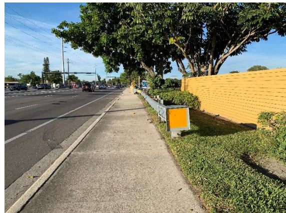
Existing guardrail to prevent trespassing by the South Florida Water Management District (SFWMD) C-13 on the eastern side of NW 31 st Avenue.
