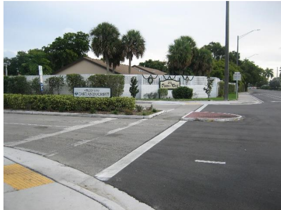
The Oakland Forest driveway provides a marked crosswalk and a median nose.
