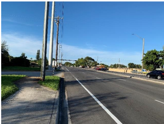
Provide an unobstructed pedestrian zone to prevent fixtures blocking non-motorized users. In addition, consider meandering the sidewalk zone if there are fixed obstructions.
