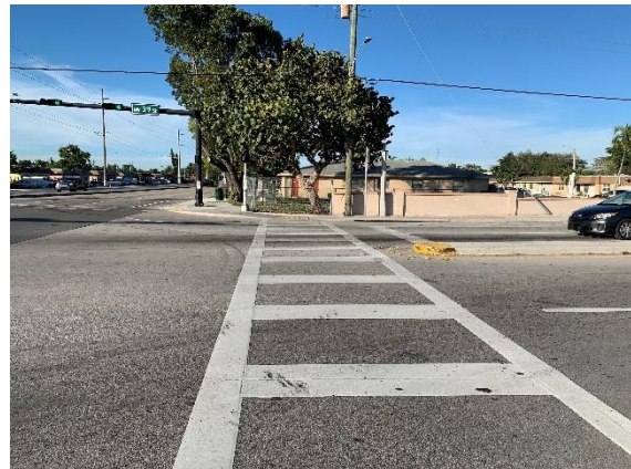
Marked crosswalk with detectable warnings on curb ramps at NW 31 st Avenue and NW 39 th Street for the northern and eastern leg.
