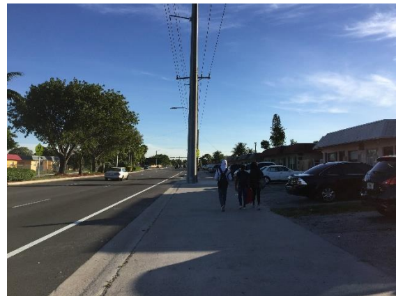
Evaluate the sidewalk condition to ensure a cross slope of 1% (2% maximum) to meet ADA standards.
