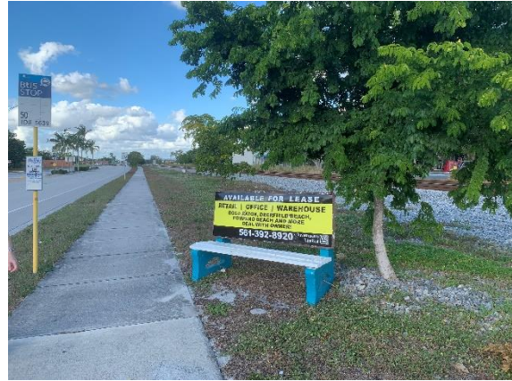
Route 50 – Stop ID# 5639 does not have ADA-compliant landing pad or shelter.
