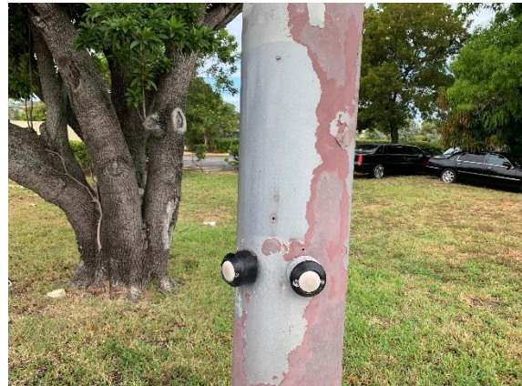
SR 811/Dixie Highway and SW 4 th Street is missing signage on the pedestrian push buttons in the northwest corner.
