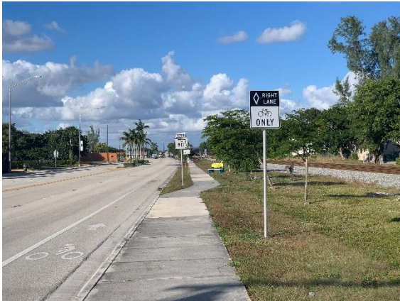
There are conventional bike lanes along the corridor with pavement markings and signage.
