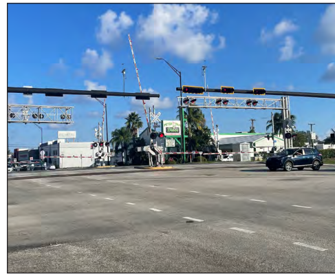
View of the intersection looking southeast
