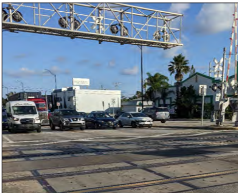
Observation 35: Crosswalk visibility issues caused by the elevation of the railroad
