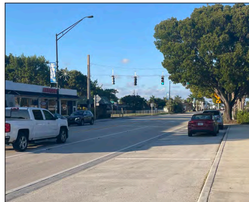
Observation 59: Large on-street parking spaces along Dixie Highway
