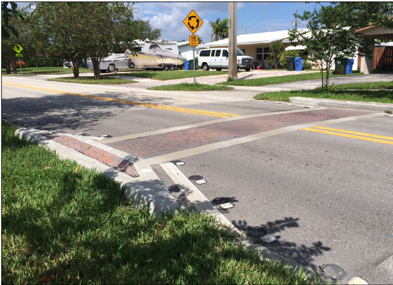
Traffic calming along NE 45th Street in City of Fort Lauderdale
