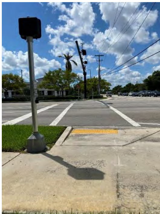
Looking south across the east leg
