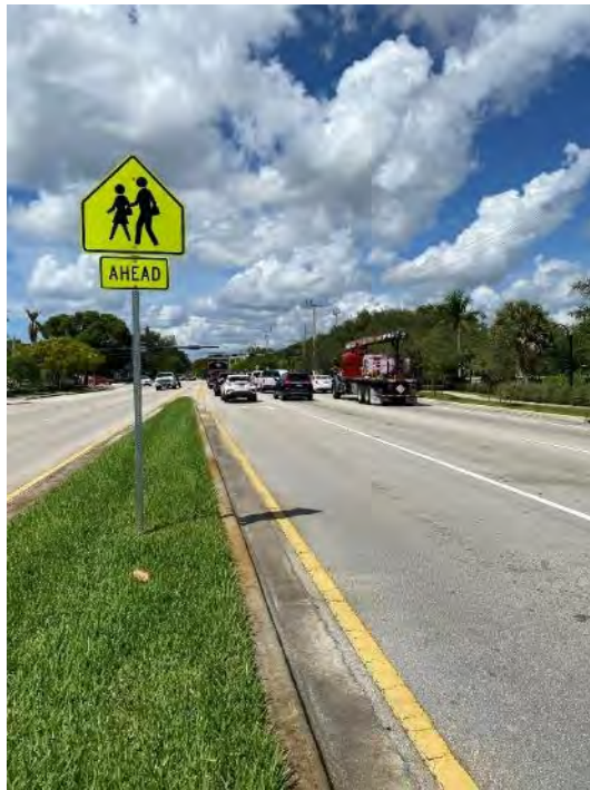
Looking west into the intersection
