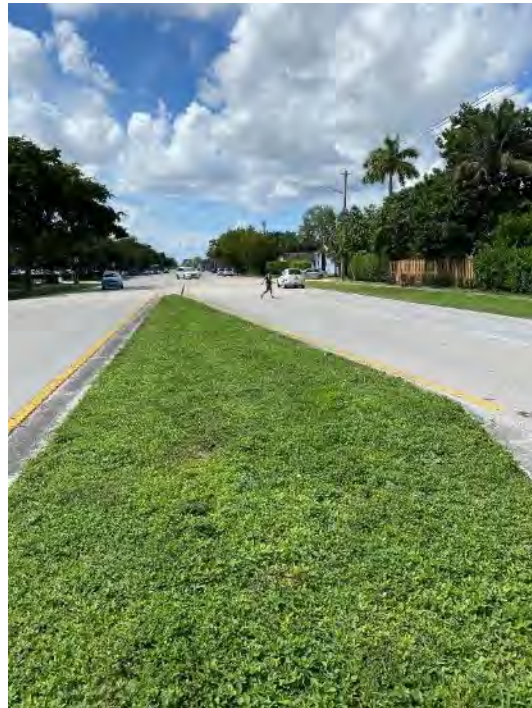
Looking west toward median opening #1
