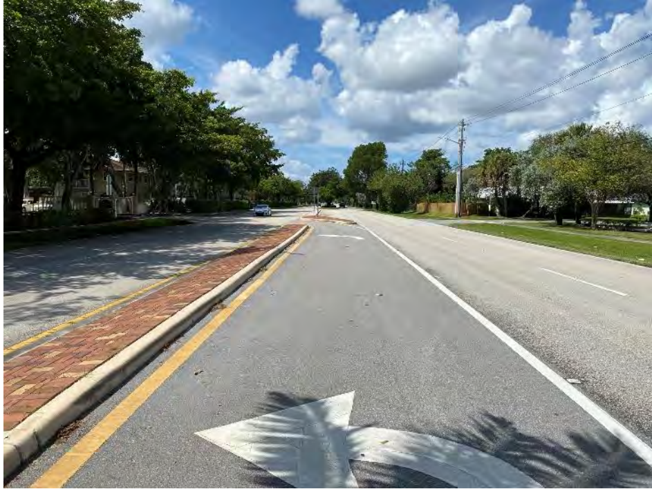
Looking west into median opening #4
