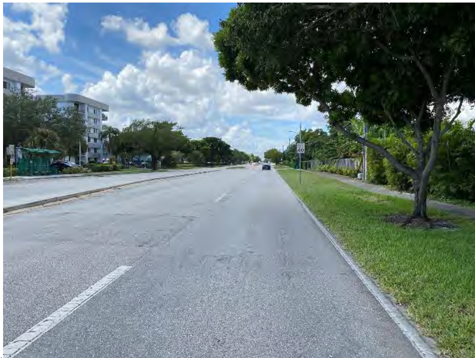
Looking west toward median opening #2
