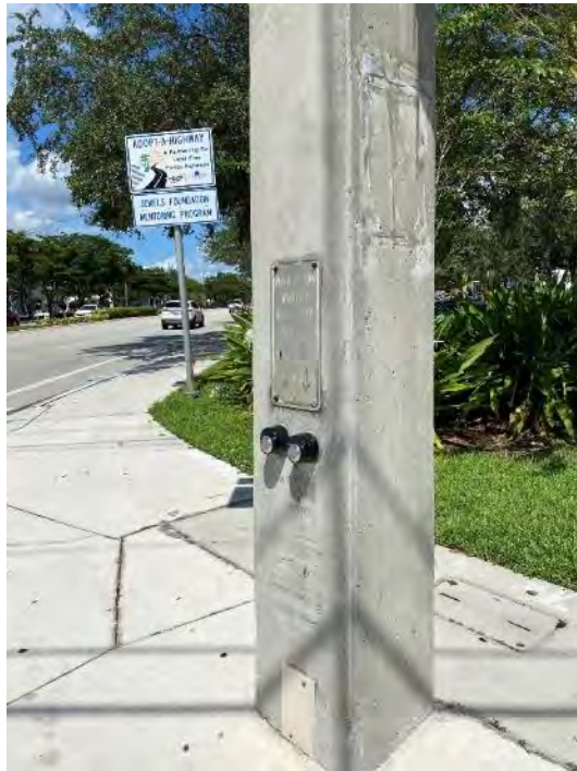
Non-standard pedestrian push buttons in the northeast quadrant at University Dr
