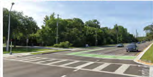
Bike Boxes + Green Pavement Markings
