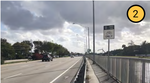
Sidewalk is between guard rail and canal with obstructions; Bike lane is only 300 ft long.
