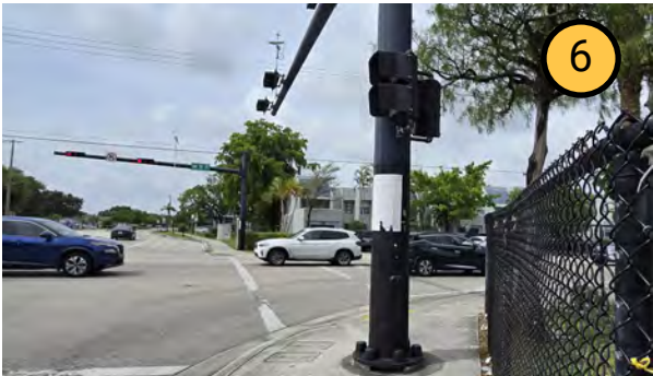
6 Mast Arm pole obstructs sidewalk in NW corner
