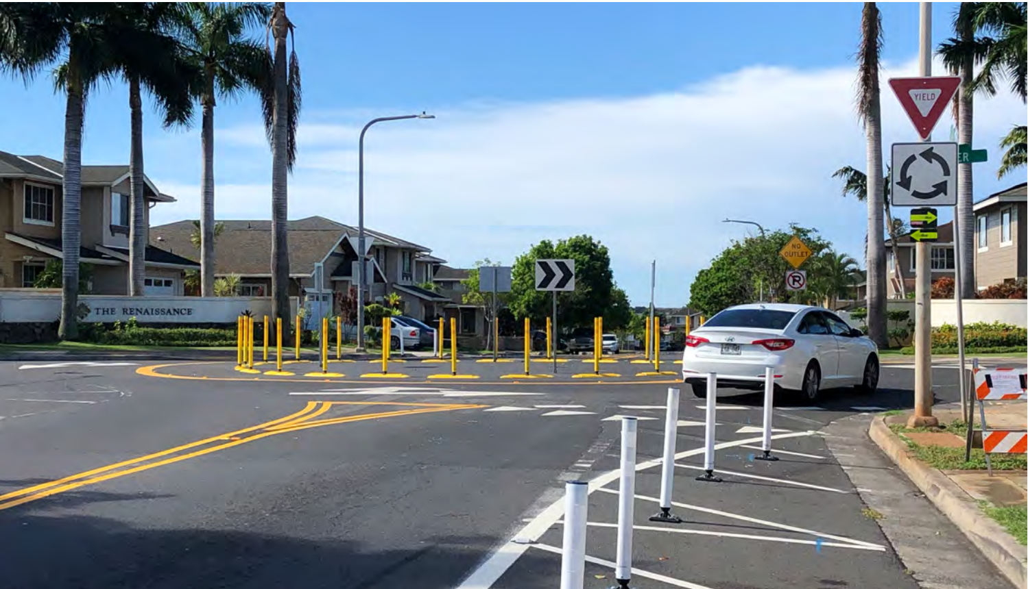
Example of a 4-way intersection converted into a Quick Build Roundabout. Low-cost materials utilized included paint, pavements markings, flexible bollards, and signage.
