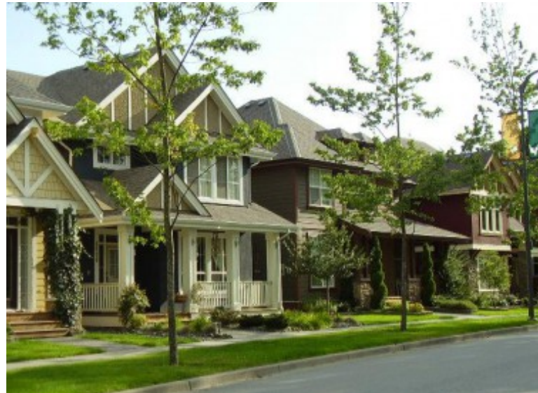
Figure 7-29: Preservation of the residential character of a neighborhood. (Image courtesy of The Fifth Estate)
