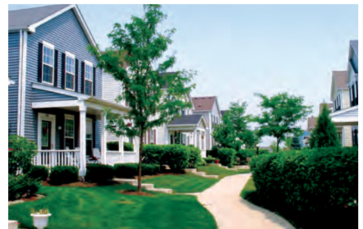
HomeTown Aurora is a 1,288-unit development built by Bigelow Homes that includes single-family detached, single-family attached, and loft-style homes. About half of the units are affordable to families earning below 80 percent of the area median income. It includes diverse housing types that appeal to a range of market segments. This compact development also combines smaller private lots with protected open space. Image courtesy of Bigelow Homes
