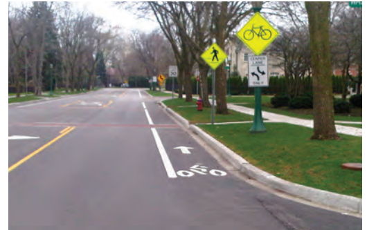
In Wilmette, an 18-month construction project has converted 4-lane Sheridan Road into a 2-lane road with bike lanes in either direction and a middle turn lane from Lake Avenue north to Westerfield Drive and the Plaza del Lago. Image courtesy of the Village of Wilmette
