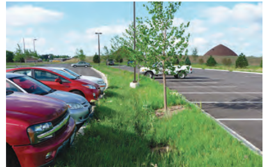
Among other stormwater best management practices, the Lake County Central Permit Facility uses native plant bioswales. These shallow excavated swales with deep-rooted native plants are designed to collect, absorb, and filter stormwater runoff and pollutants that collect on the parking lot pavement from automobiles. County government can be a leader in using stormwater best management practices. Photo and description courtesy of Lake County.
