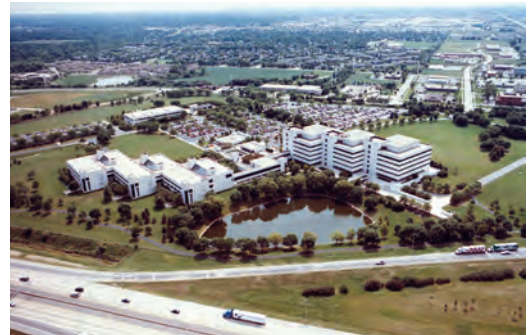
The Advanced Research Projects Agency - Energy (ARPA-E) was established within DOE to fund projects to develop technologies that reduce energy related emissions and improve energy efficiency. Nalco Company, based in Naperville, received $2.2 million to capture and desorb carbon from smokestacks of coal-fired plants. Image courtesy of Nalco Company
