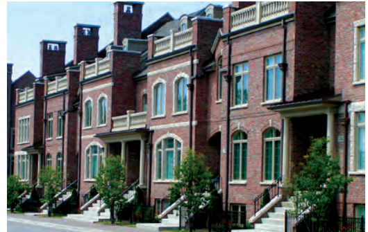
In Palatine, a brownfield site near this residential development was redeveloped as structured parking as part of a larger downtown development effort. The cleanup had significant catalytic effect on nearby properties as well, with the value of nearby property doubling within five years after completion of the cleanup. Image courtesy of Patrick Barry
