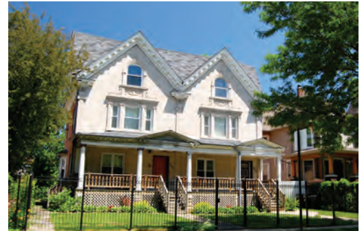
The Village of Oak Park used federal Community Development Block Grant (CDBG) and Home Investment Partnership Program funds from HUD to fund a single-family rehabilitation program. The program serves low and very low-income homeowners by helping them maintain their homes at safe and desirable standards while preserving the Village's housing stock. Image courtesy of Eric Rogers
