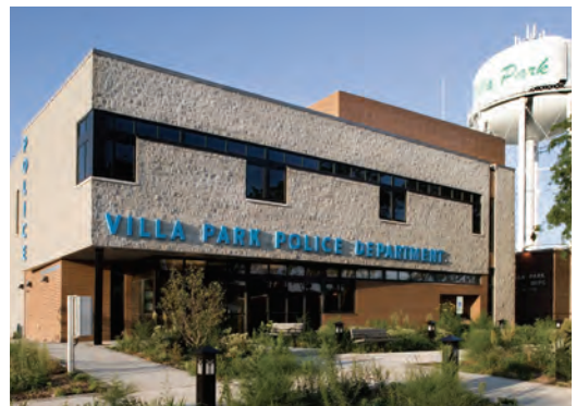
The Villa Park police station in DuPage County was built on the site of a parking lot downtown. It decreased runoff in its mostly built-out watershed by three stormwater best management practices: a green roof, bioretention swales, and permeable paving in the parking lot. The police station is also an example of infill development. The project was partly financed by a grant from the Illinois Environmental Protection Agency (IEPA). Image courtesy of IBC Engineering Services, Inc.
