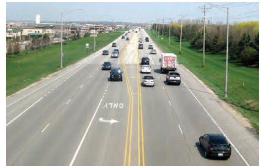
Kane County is working in partnership with a group of municipalities to improve transit accessibility along Randall Road for Pace Route 529. The existing corridor lacks sufficient access for pedestrians and disabled persons, while many of the buildings along the corridor have large setbacks with extensive parking, limited sidewalks, and no waiting areas. The study is intended to address these design issues across the five municipalities in the corridor (Aurora, North Aurora, Batavia, Geneva, and St. Charles). Image courtesy of Flickr user geonerd
