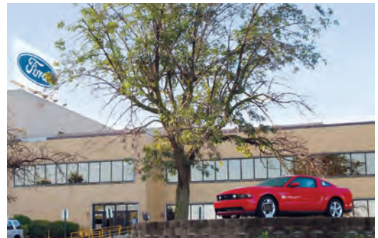
The Ford Motor Company Stamping Plant in Chicago Heights retrofitted its lighting systems with the help of the ComEd Smart Ideas incentive program. Ford replaced more than 1,000 lighting fixtures with high performance, energy efficient models that use 50 percent less energy than the old fixtures and have a longer life. Ford also installed sensors to turn off lights when personnel were not using the room. Image courtesy of ComEd
