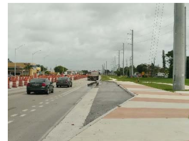
FIGURE F-2 (RIGHT): NEW BUS PULLOUT ON SOUTHBOUND SR7 SOUTH OF HOLLYWOOD, AWAITING SHELTER INSTALLATION
