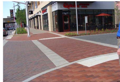
Raised Pedestrian Crosswalk
