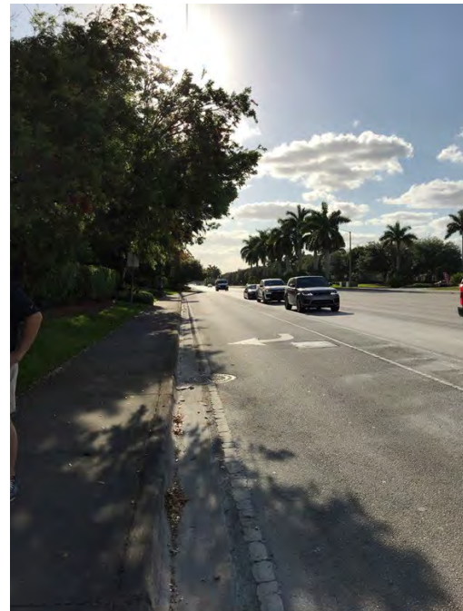
Observation 14: “No light poles on south side.”
