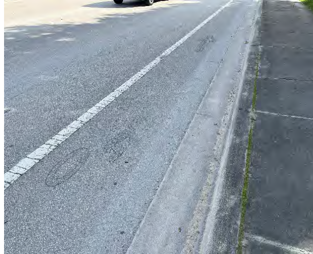
Bicycle lane striping along the south side of Miramar Parkway is now worn away and hard to discern.
