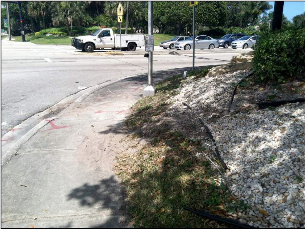
Photo 22: SE Corner of Lyons Road and Copans Road, Sand Dangerously Spilling onto Sidewalk
