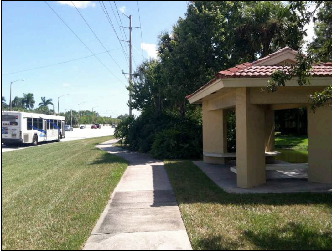
Photo 21: Privately Constructed Bus Shelter, Not Aligned with Bus Stop
