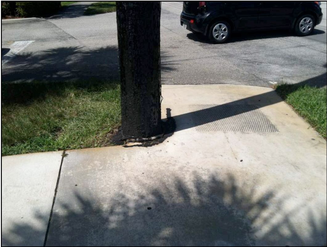
Photo 27: Wooden Utility Pole with Black Tar Covering It
