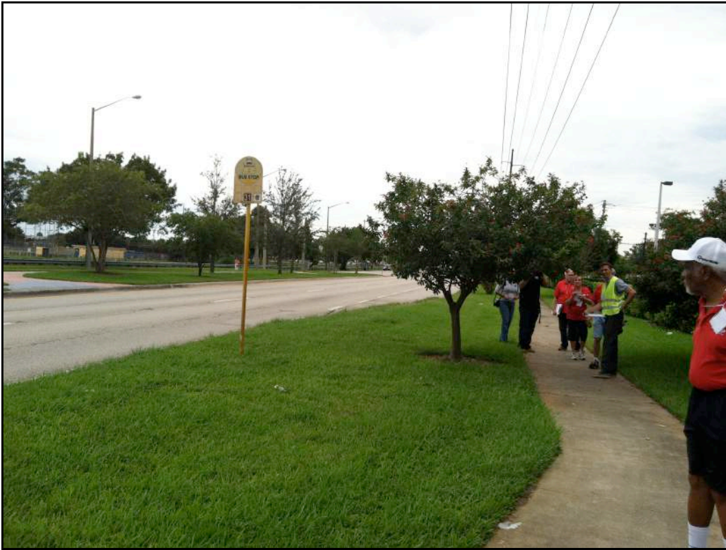
Photo 06: Bus Stop Without Amenities or ADA Landing Pad, East of Lyons Plaza
