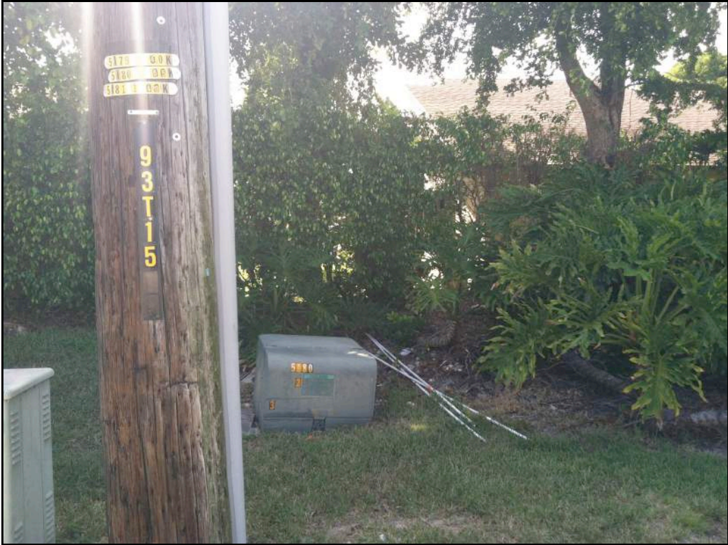
Photo 13: Example of Construction Debris on the Side of the Road, West Side of Lyons Road
