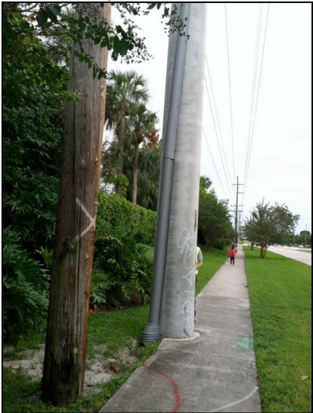
Photo 08: Utility Pole within the Sidewalk Path, on West side of Lyons Road
