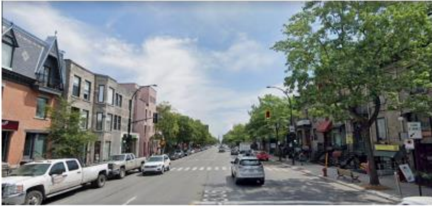
Saint-Denis prior to road treatment
