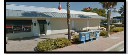
Sidewalk Surface Treatments
